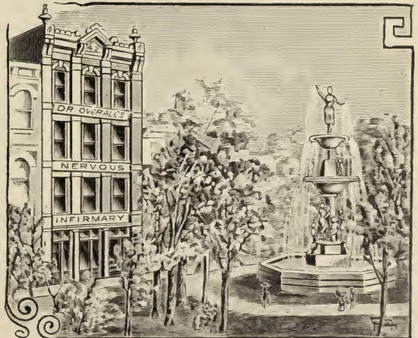
DRS. OVERALL & PEETE'S INFIRMARY. North Side Court Square.
